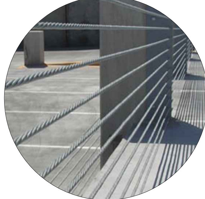
7 42" H. CABLE CRASH WALL (HORIZONTAL WIRE SHOP DRAWINGS TO BE APPROVED PRIOR TO INSTALLATION)
